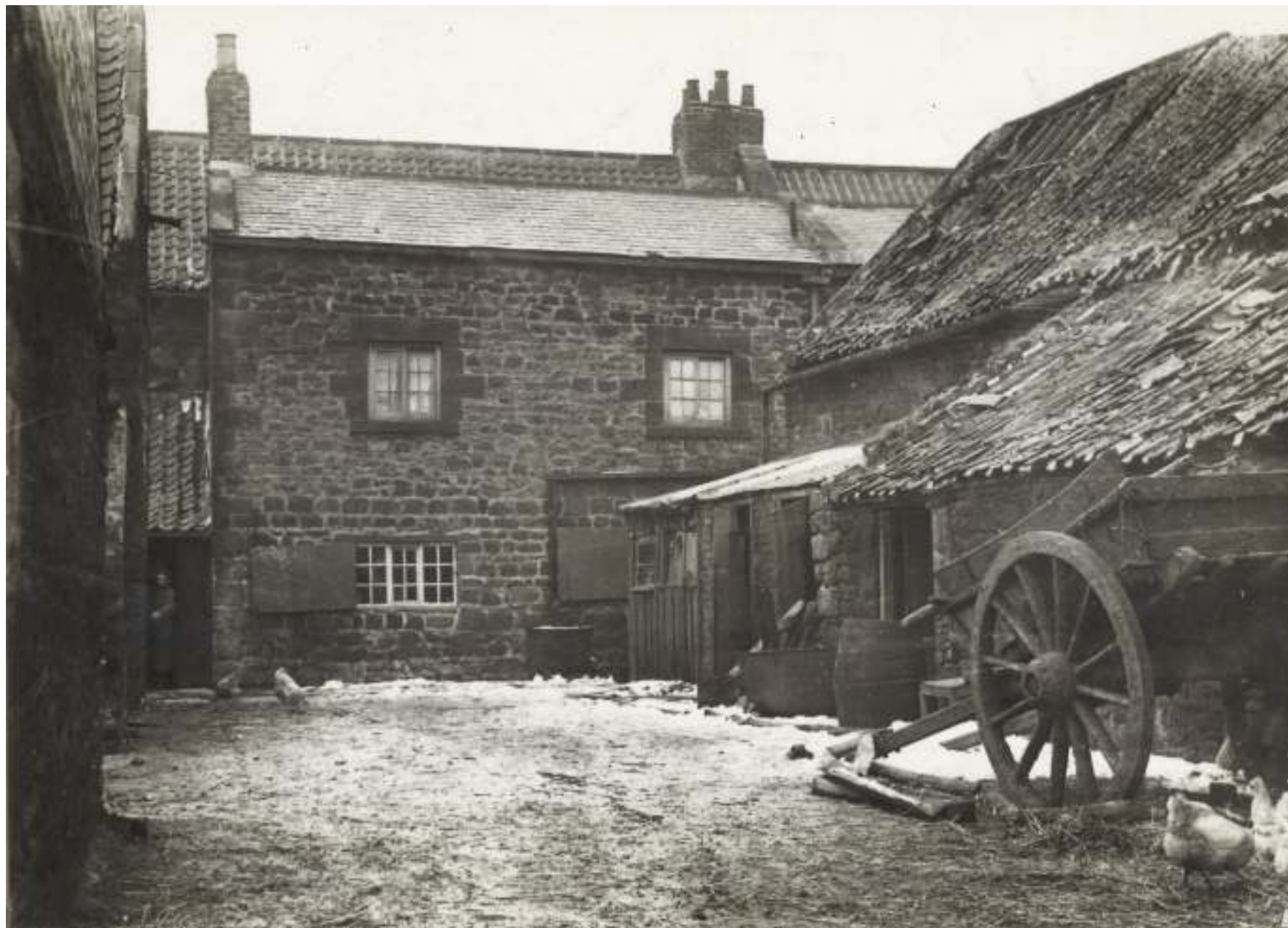
Fig. 11: Part of the yard of East Farm, showing the back range of the farmhouse (Building 12) and lean-tos against Building 13 (note missing roof tiles). c.1925, winter. Newcastle Library Local Studies (Newcastle/agriculture/farms/Walker East Farm).
