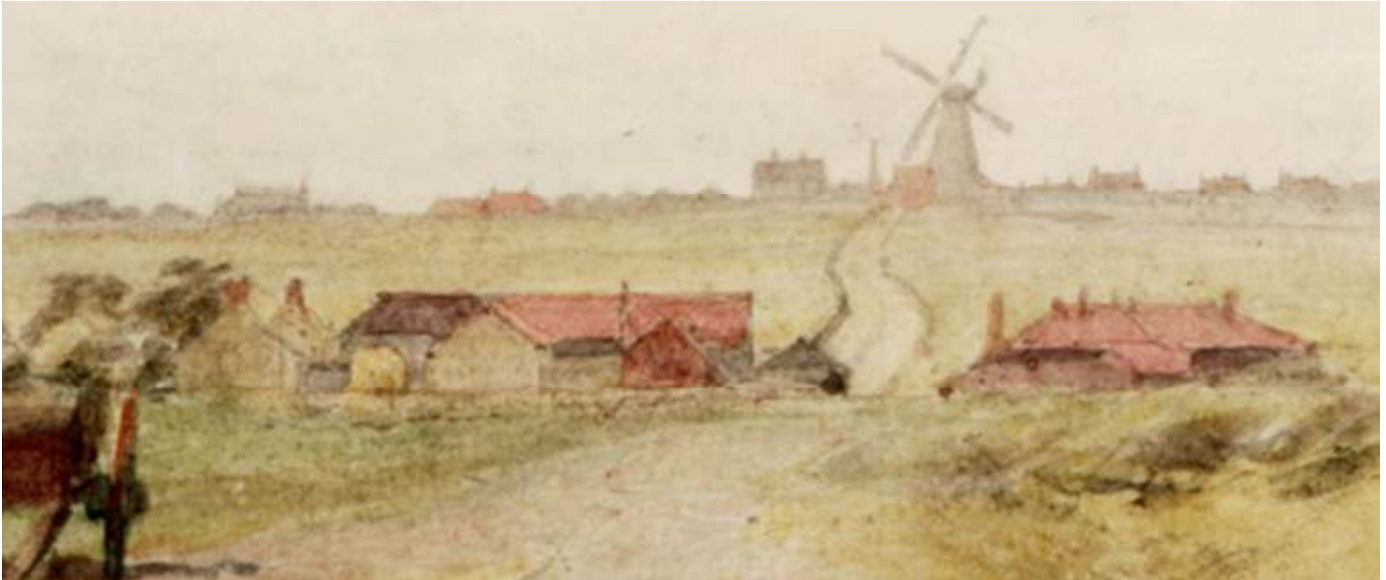
Fig. 6: Detail from Richardson's watercolour of Stott's House Farm, showing East Farm from the east in 1848. To the left is the roofless stone building. The building with the brown roof may be the gin-gang (Building 9), with a straw-stack in front of it; the stone-built gable end is the original farmstead (Building 7). Behind are the pantile roofs of Building 13, showing the division in the roof still visible in Fig. 12. The red gable end is Building 5, and the grey gable end Building 1. To the right of the road are miners' cottages related to Gosforth pit. TWCMS : G3851.
