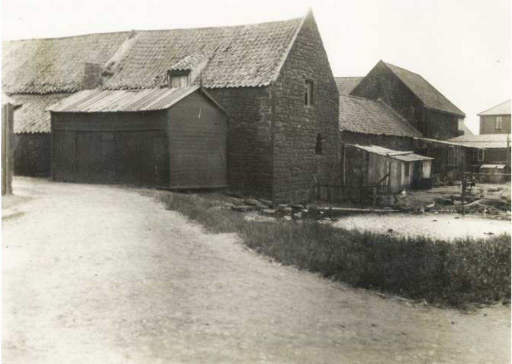
Fig. 12: Walker West Farm from the entrance gate into East Farm, showing Building 13 (behind the wooden hut), with nos 14 and 15 behind, and the duck pond, 1933: Newcastle Library Local Studies (Newcastle/agriculture/farms/Brown's farmstead)
