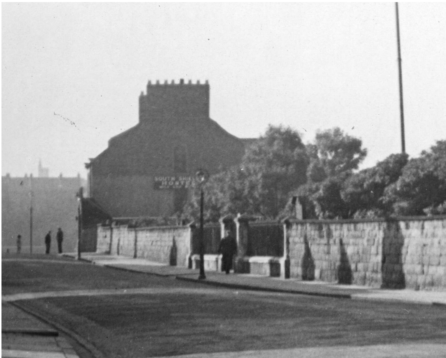
Fig. 25. Detail from a photograph of Mile End Road showing Mile End House from the south. There are two central windows, a 'Hostel' sign, and a change in the colour of the bricks; this side once had the ropery built against it. The roof of the wing projecting from the front of the house is partially visible behind the trees. Photographer A. Flagg, July 1937. © South Tyneside Libraries.
